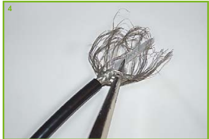
Using the pointed tool, carefully unweave the braid strands.
