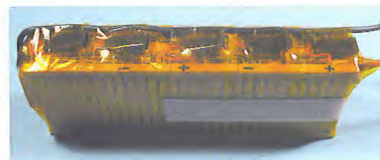
Figure 13. Extra connections are brought out to allow the individual cells to be monitored.
