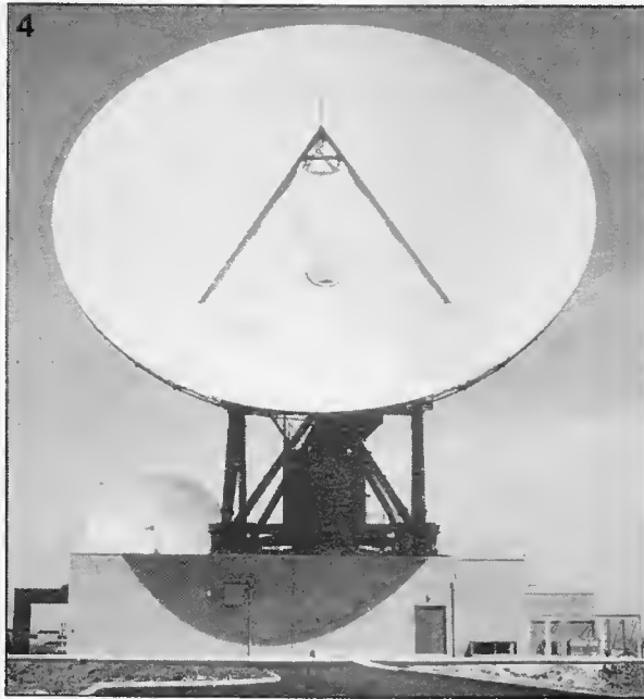
Fig. 4. Aerial 6 is Goonhilly's largest dish with a diameter of 32 m. It was also the first "dual frequency" antenna, able to transmit and receive on two different frequencies simultaneously. Photograph courtesy of British Telecom.
