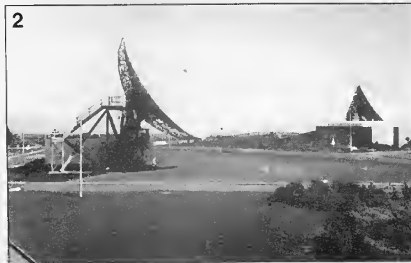
Fig. 2. A small section of Goonhilly Downs Earth Station: in the foreground Aerial No. 7. Photograph courtesy of British Telecom.
