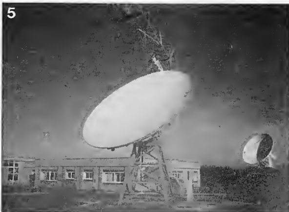
Fig. 5. The latest of the antennas (No. 10) to be installed at Goonhilly Downs. Photograph courtesy of British Telecom.
