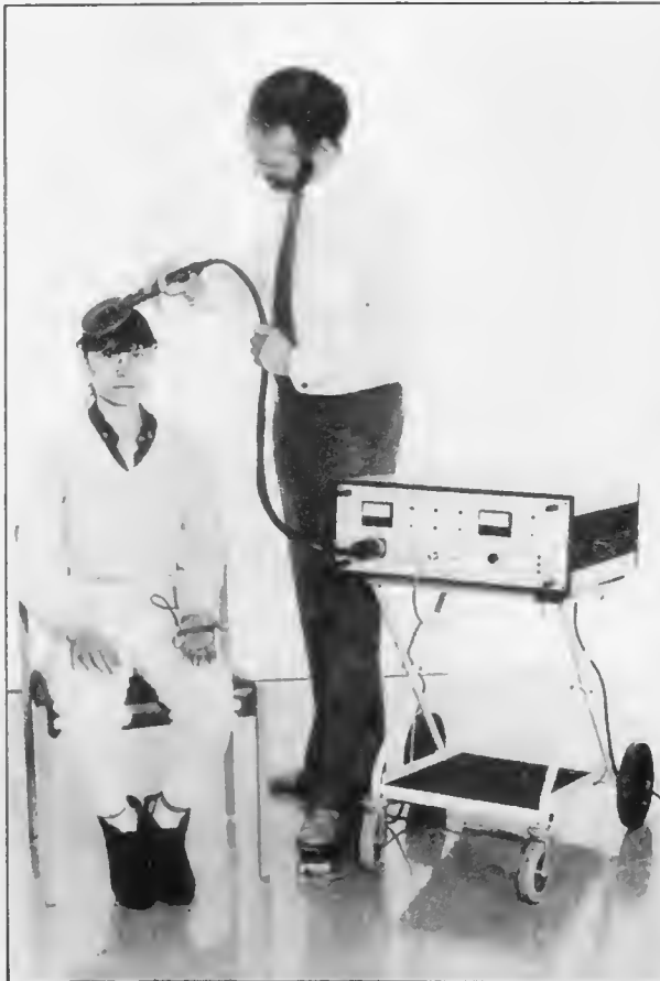
The prototype magnetic stimulator in use.
