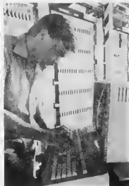
Checking System X with the aid of a visual display terminal.
